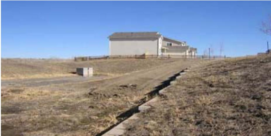
**Figure 5: EDB with Access Road and Rock Around Outlet Structure**
