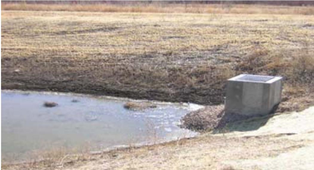
**Figure 7: EDB with Micropool & Rock Outlet**
