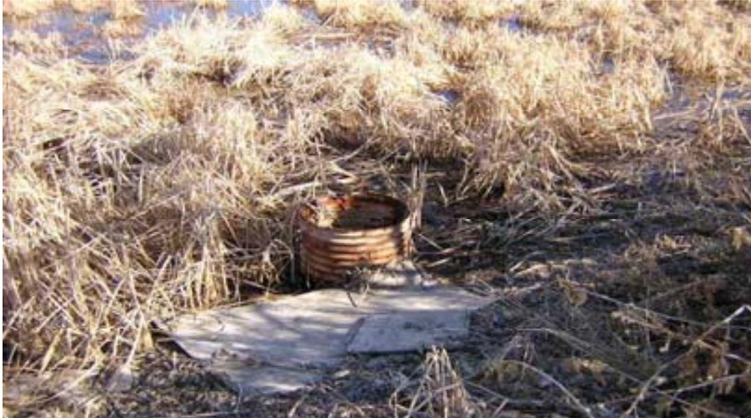
**Figure 9: Outlet Structure of Perforated CMP Culvert**
