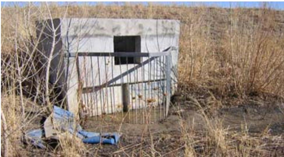
**Figure 6: Outlet structure with heavy siltation, preventing drainage**
