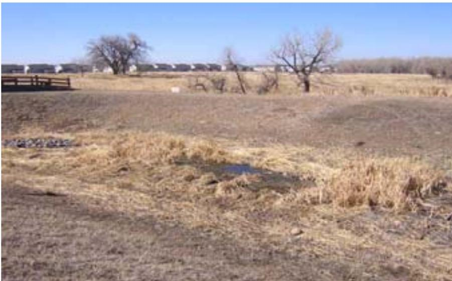
**Figure 4: Extended Detention Basin, with “Permanent Water” and Wetland Vegetation**
